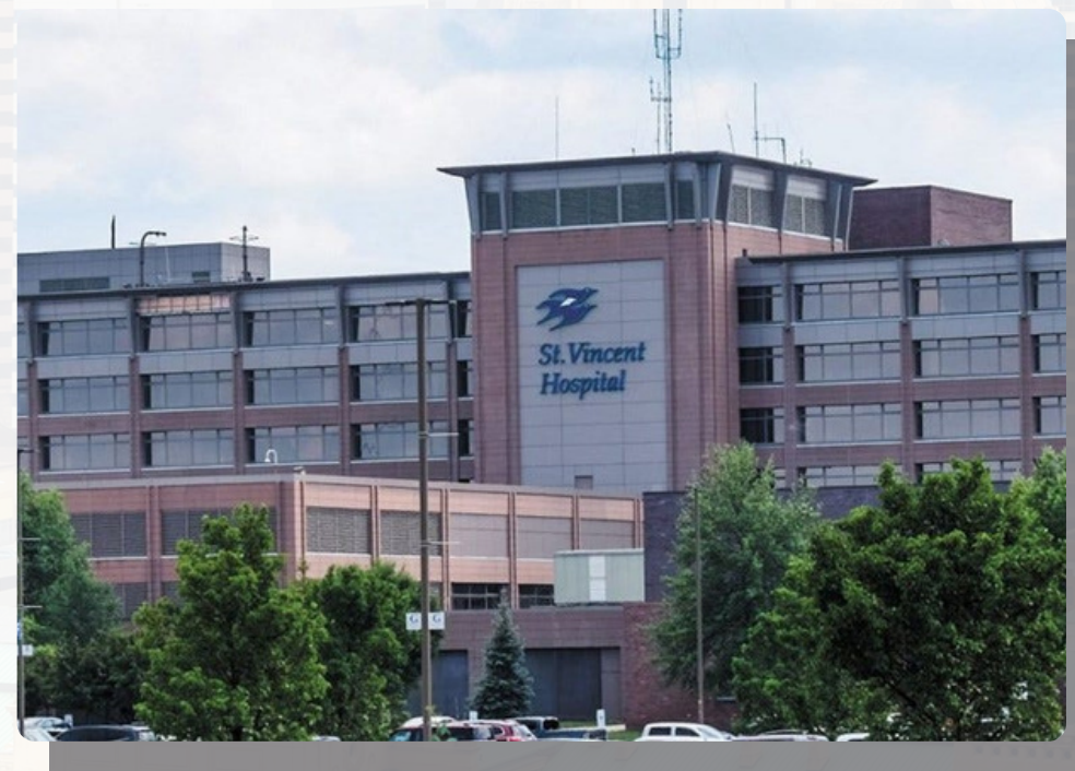
Ascension St. Vincent Hospital
